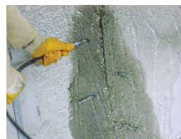
Hose set coupling to installed mechanical packer.
