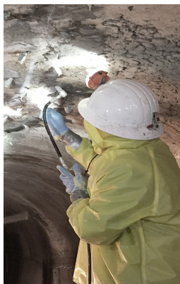
Over Head Injection with Button Head Packers
