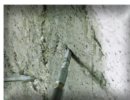
Packer placement, staggered, at 45 degree angle.
